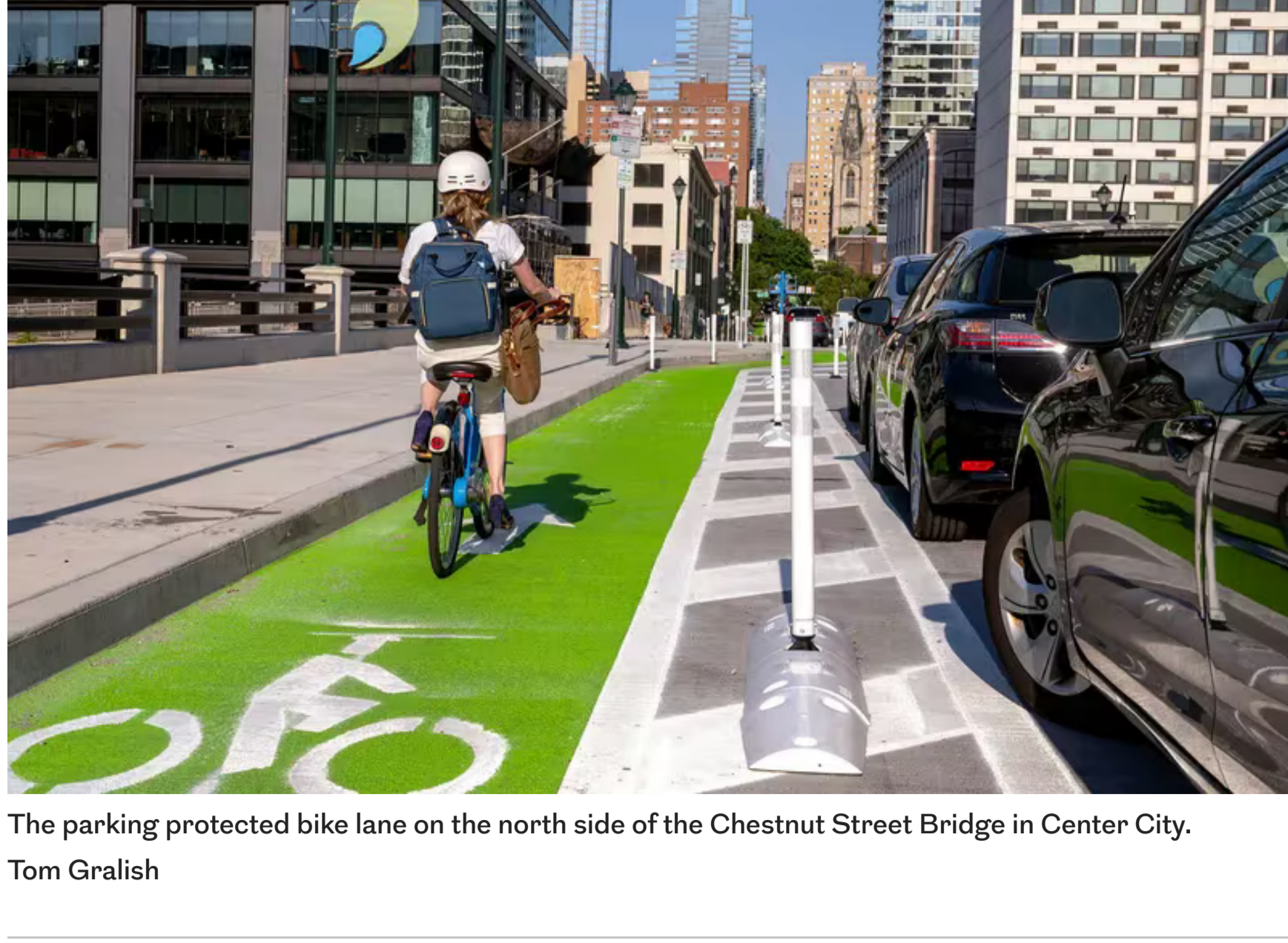
The parking protected bike lane on the north side of the Chestnut Street Bridge in Center City.
