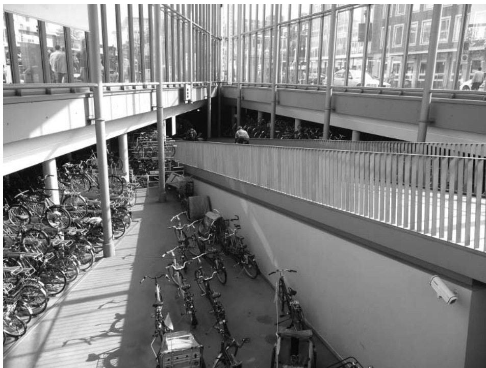
Figure 18. Deluxe parking for 3,300 bikes at the main train station and bus terminal in Muenster, Germany. The bike ramp connects the street level to the bike parking level, from which there is direct access for cyclists to all train platforms. All bus stops are at ground level just to the left of the bike station.
