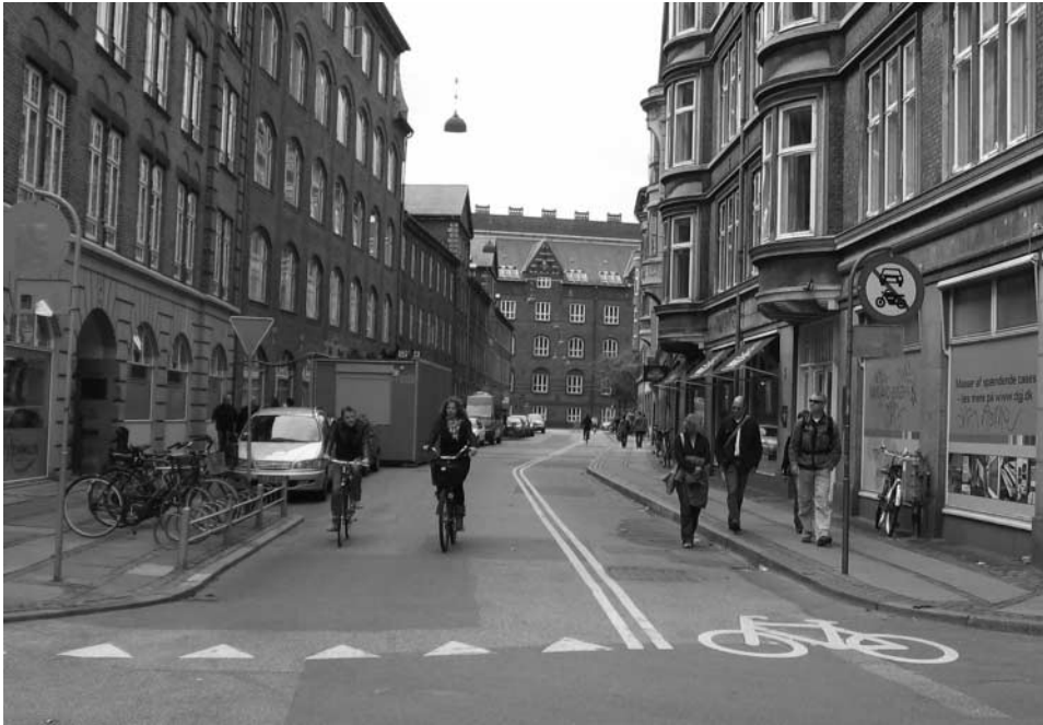
Figure 15. This contra-flow lane in Copenhagen enables cyclists to ride in both directions, while cars are restricted to one direction. The roadway has been deliberately narrowed through the provision of bike parking. In effect, these modifications have turned it into a bicycling street, where cyclists outnumber motorists.
